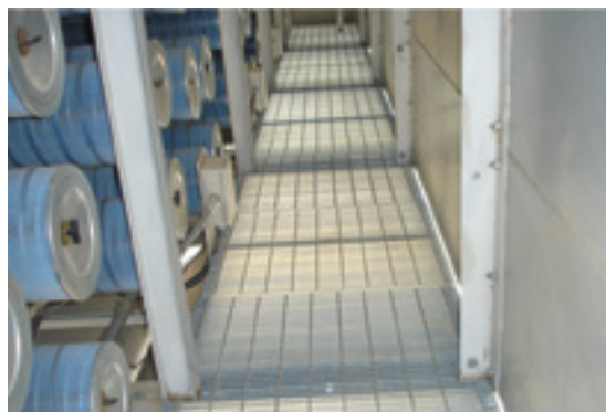
Inlet filter house floor , originally made of steel plate, was replaced with steel deck grating to prevent snow drifting in winter which blocked air flow and to eliminate a slip hazard. Beatrice Power Station
