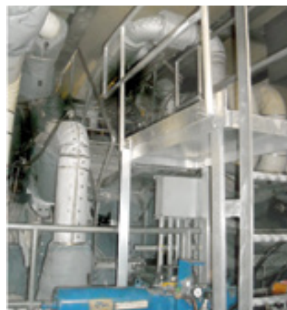
Permanent platform provides safe access to gas-turbine igniters. Granite Ridge Energy
