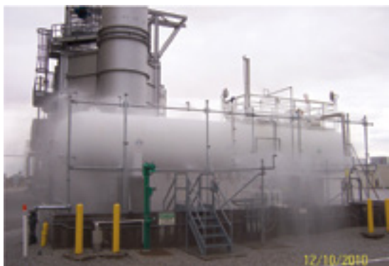
Ammonia-tank leak-suppression system protects plant personnel and neighbors. Water spray system, which has 34 nozzles configured on six lines surrounding the tank, was designed to NFPA
