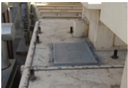
Roof hatch over bearing tunnel facilitates confined-space rescue. Edward W Clark Generating Station
