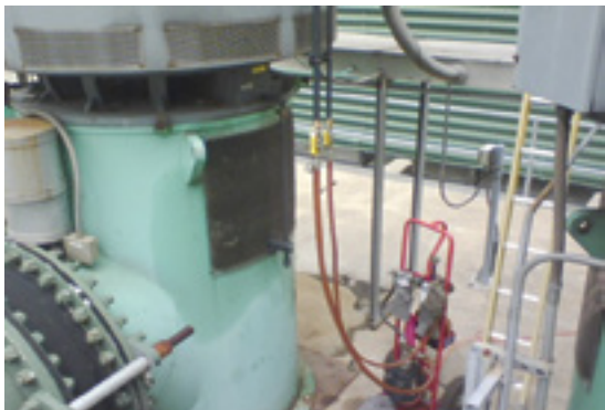
Mobile filter cart and piping modifications allow ground level access to circ-water-pump motor lube sump making hazard-free a job that had been dangerous. Allegheny Energy Units 3, 4, 5
